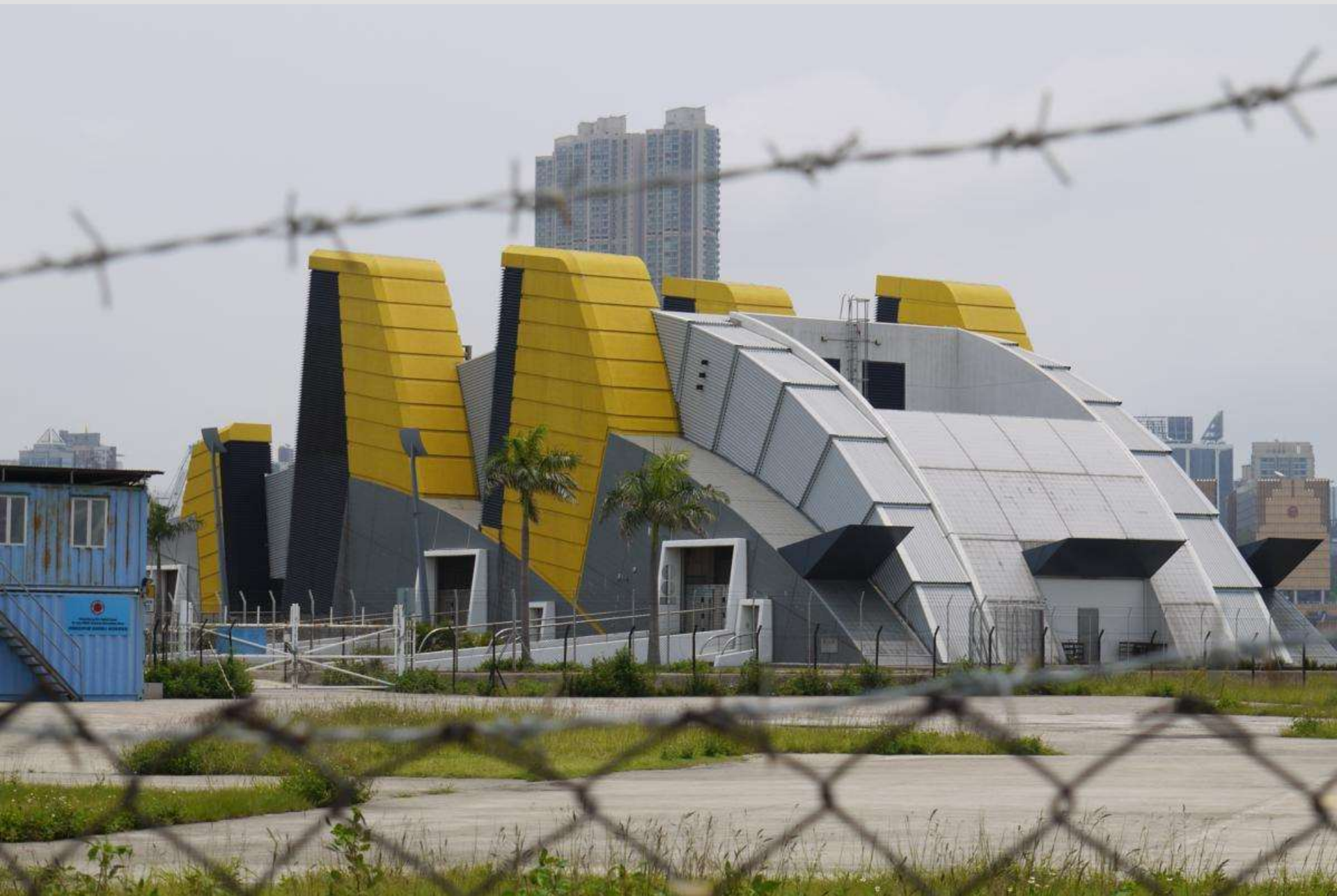
Ventilation Building of Kowloon Station, Hong Kong
